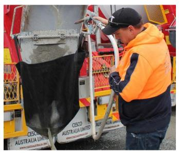
**STEP 3** - Use the mixer truck hose to wash gravel, sand and cement residue into the Washout Warden.
