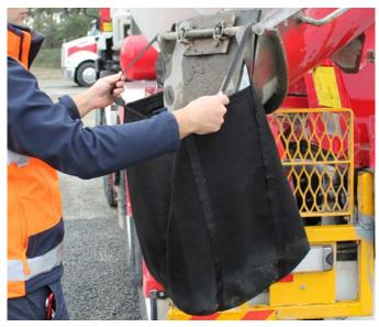
**STEP 1** - Place the Washout Warden over concrete mixer chute pins.
