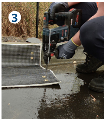
Using the GuardDog eyelets: a) Drill and secure with concrete screws OR b) use plastic or metal ties to secure to the drain grate.
