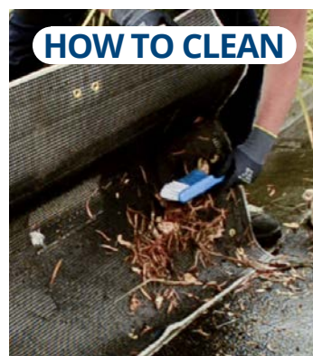
a) Use a brush or broom to sweep away leaves and debris. b) Can also be hosed from behind to remove silt build up.
